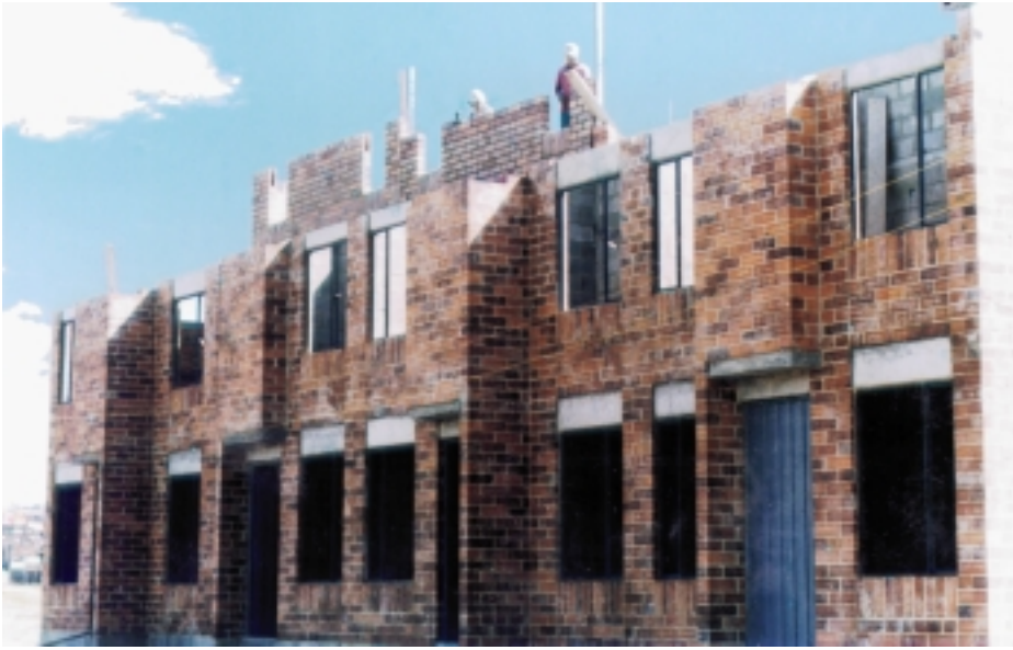
Left: Walls made of fair-faced clay bricks and hollow blocks
