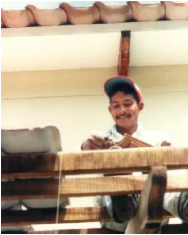
Above: The roofs are covered with Micro Concrete Tiles
