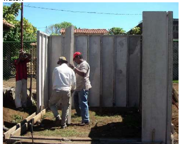
Assembly of ferrocement panels for a core shelter
