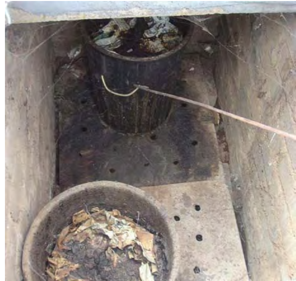
Servicing: the "dry bucket" is lifted out with a hook and its content used as fertilizer or disposed
