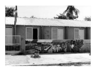
In the Dominican Republic MCR roofs did not suffer while zinc roofs were severely damaged and the vaulted brick roofs were not affected.
