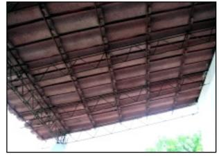
The picture above shows a bar structure (it is important to highlight that it was made in a factory and is of unusually good quality): The beams are placed at a distance of 75cm and bars of 3/8" are used as battens. These bars deform with the weight of the tiles and the finished roofs is irregular. This solution becomes more expensive than using Csection and tubes.
