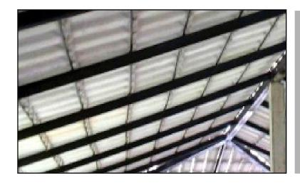
This picture clearly shows deficiency of the bar battens. Even on beams of «Csections", it is difficult to obtain straight lines, apart from the fact that the weight of the tile makes the bar bend.
