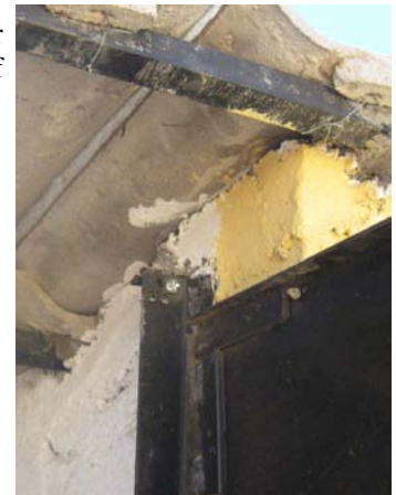
south door roof
