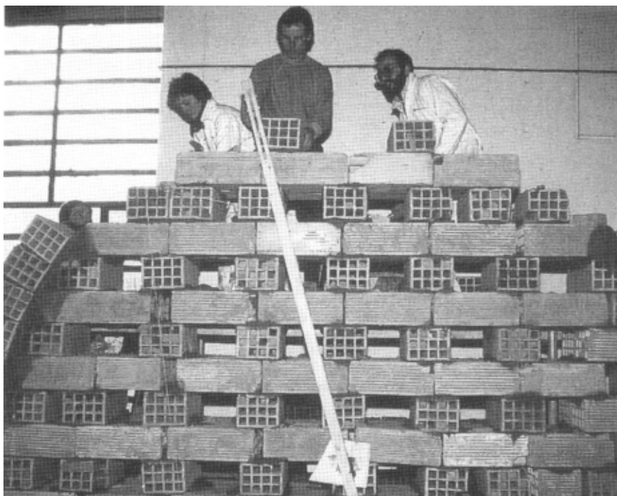
Brick formwork
