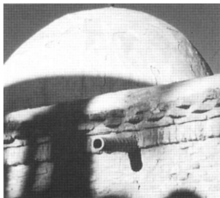
Ensuring water run-off through a water-spout
