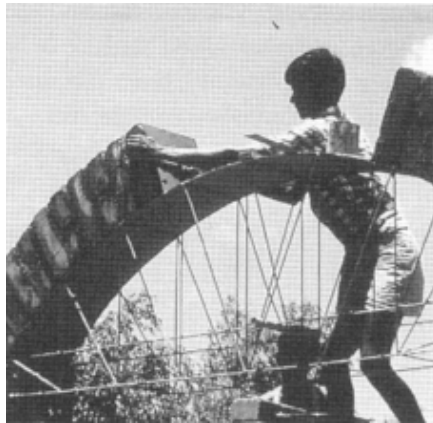
Metal formwork
