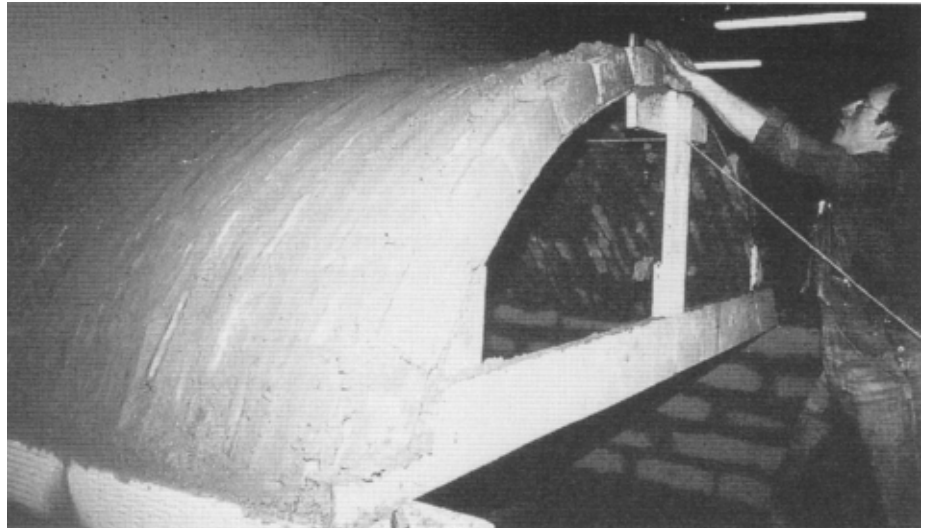
Building a barrel vault in "slices"
