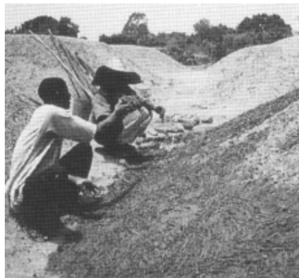
Earth plaster is efficient but often requires maintenance
