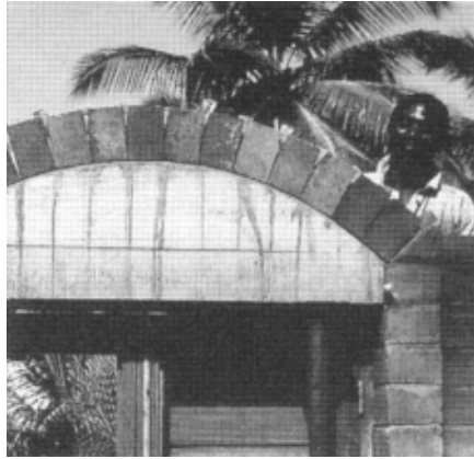
Wooden formwork
