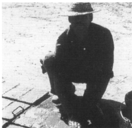
Moulding an adobe block into the shape and size required
