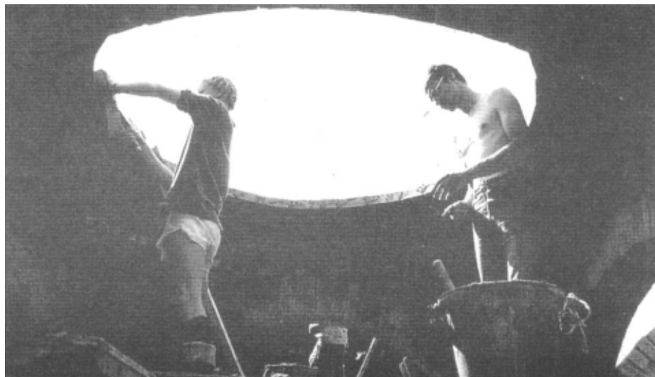
Building a cupola using inclined ring-courses
