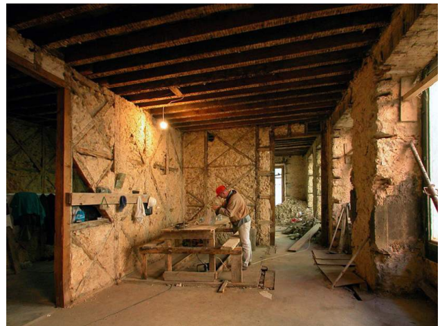
Insight into restoration of a gaiola (Foto R. Langenbach)
